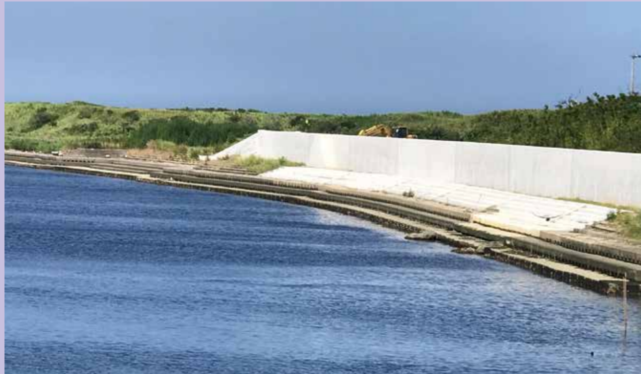
Construction to raise the banks of Ichinomiya River
