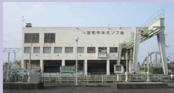
Ichinomiya Town's Main Drainage Facility
