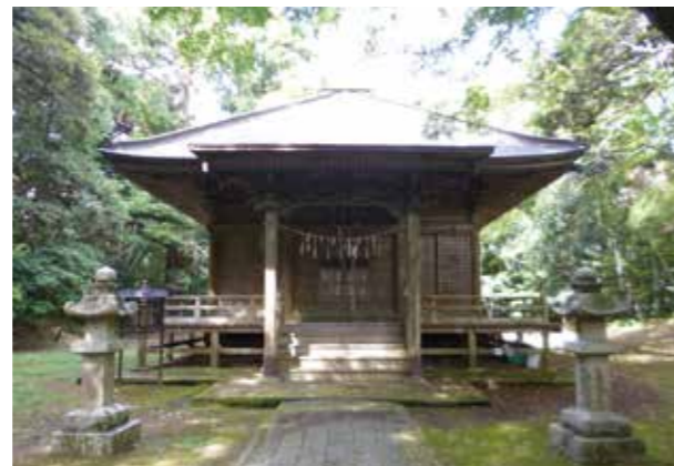
Torami Temple's Main Hall [designated tangible cultural property of Ichinomiya Town] built in 1723.
